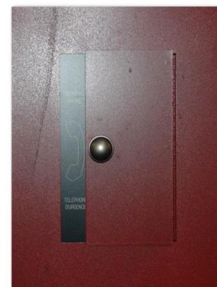
ALL other Areas of Refuge NOT fitted with the Red Firefighter phones is fitted with a yellow Emergency Phone; these are 2-way voice communication call box that is a direct connect to Campus Security Services, 24x7:
