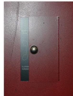
ALL other Areas of Refuge NOT fitted with the Red Firefighter phones is fitted with a yellow Emergency Phone; these are 2-way voice communication call box that is a direct connect to Campus Security Services, 24x7:
