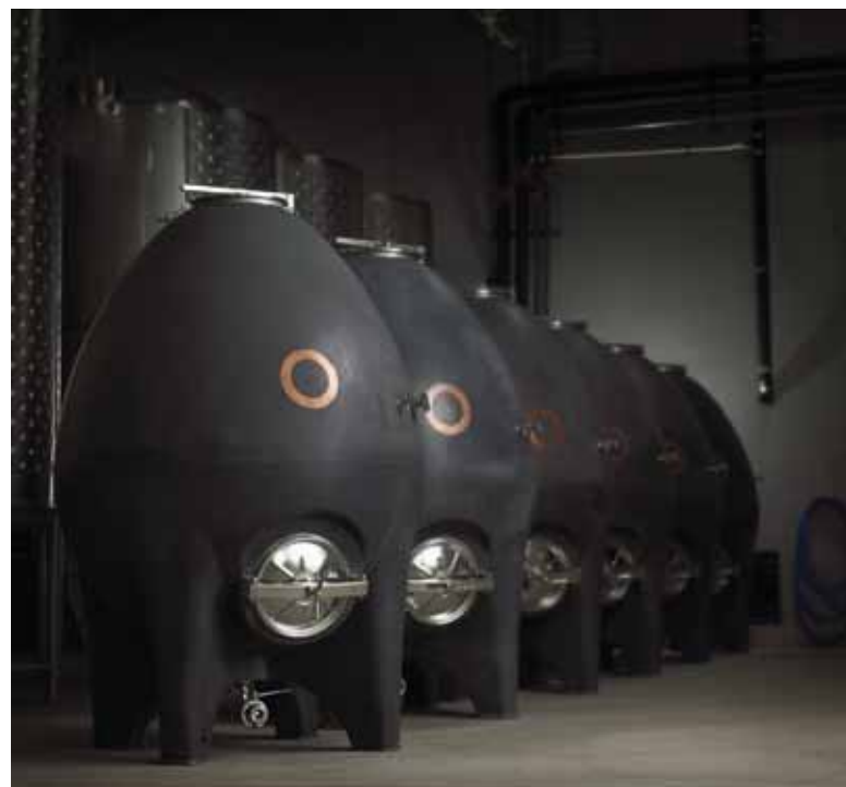
Six egg-shaped concrete tanks have been installed for fermentation. Photos courtesy of Okanagan Crush Pad.
