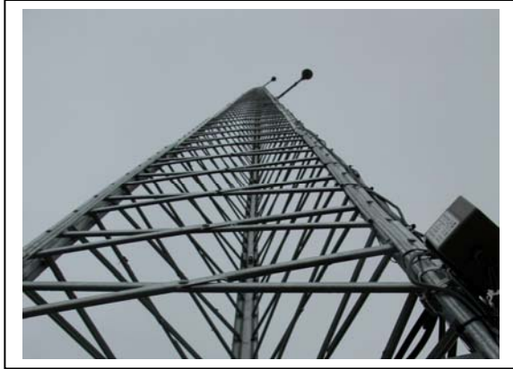
Figure 13: A 20 m (66 ft) tower lets researchers monitor air temperatures from vine level to the top, plus wind speeds in real-time over the Internet.
